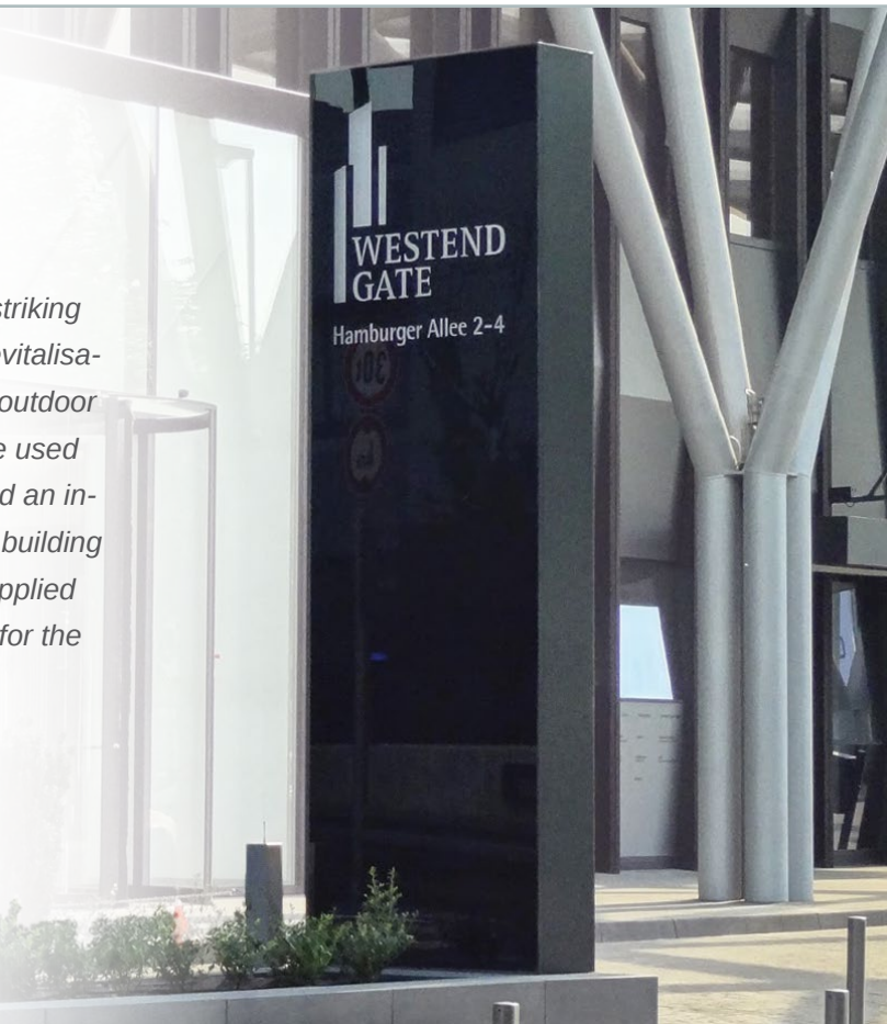
Pointing the way in the truest sense of the word: the columns around the WestendGate. They rise up to 4.10 metres, are 40 centimetres deep and between 1 and 1.5 metres wide. They were developed by unit-design and manufactured and installed by Arnold.
